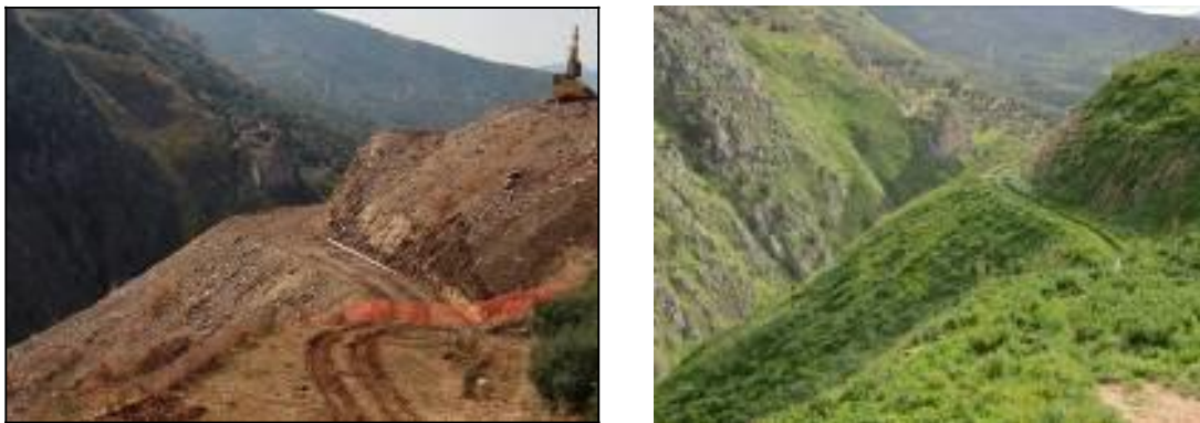
Figure 2. Case study of a 20000 m 2 slope landfill in Sicily (PA): before and after installation of the DRP solution (Solution 3, in Figure 1).
